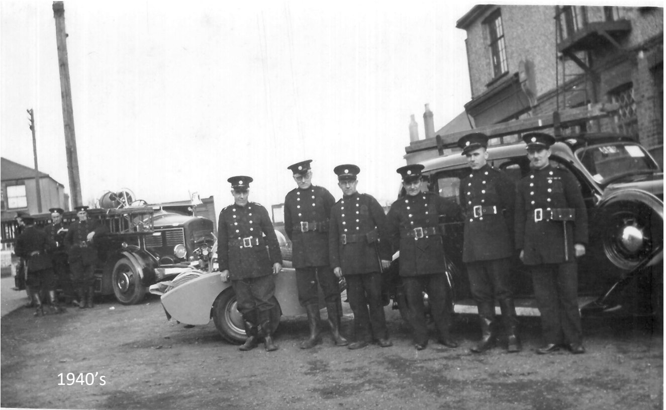
Out side of Vange Fire Station
